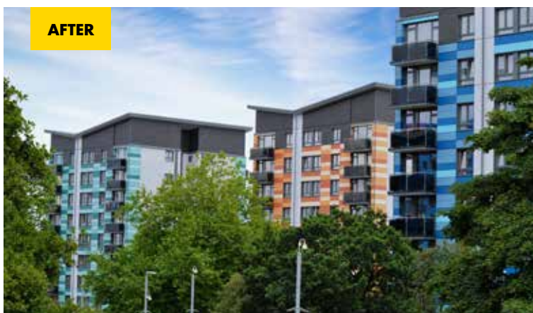
RECLADDING CHARLEMONT FARM ESTATE, UK.
