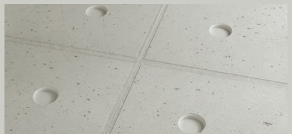
Formwork 02 mit umlaufendem Falz Formwork 02 with continuous rebate
